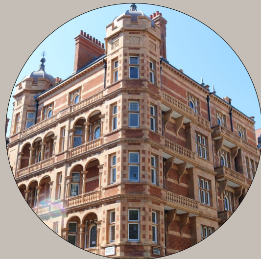
Retained Façade 1-7 Harley Street
