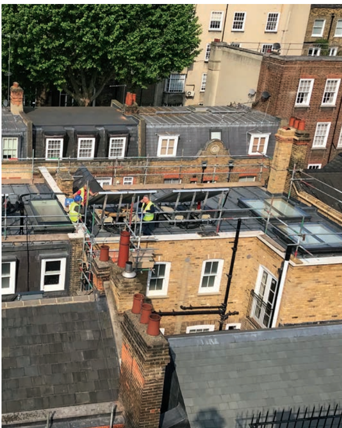
Wigmore Place, roof mounted solar panels
