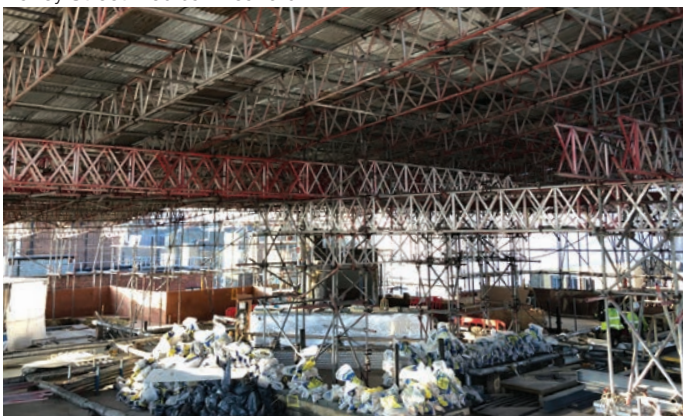
Refurbishment at Stone House, 9 Weymouth Street
